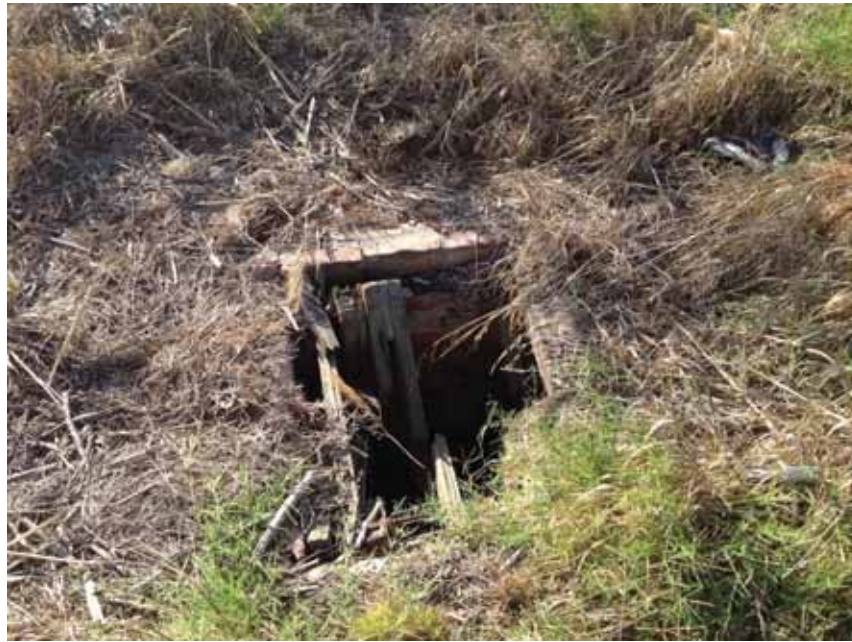
Photograph 3 Abandoned buried structure typical on north west of site near Amec Foster Wheeler soil boring B-1. Groundwater observed at approximately 4 feet below ground surface. (10/06/2015)
