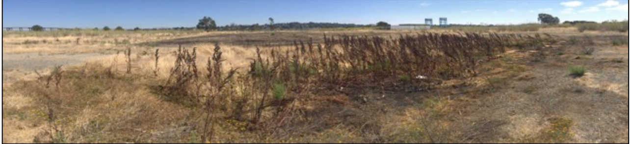
Ruderal uplands growing through eroded asphalt.
