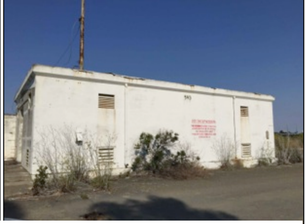
Photo 2: One of many buildings available for use by bats.
