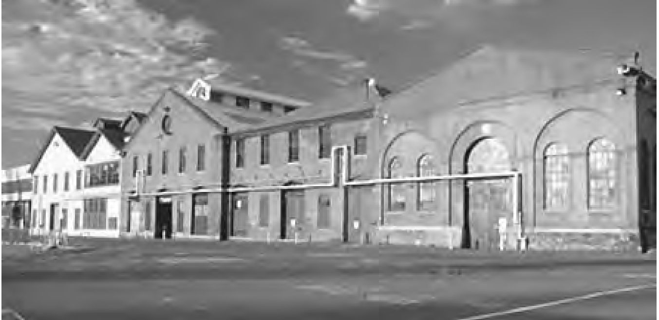
Smithery Building (Right) and Industrial Shops along California Avenue
