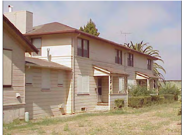
Building 0376A (Enlisted Quarters, 1941)
