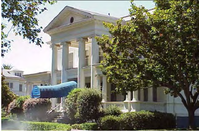
Building A (Officer's Quarters, 1900)
