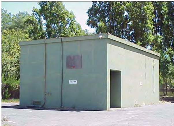
Building 0671 (Electrical substation, 1942)
