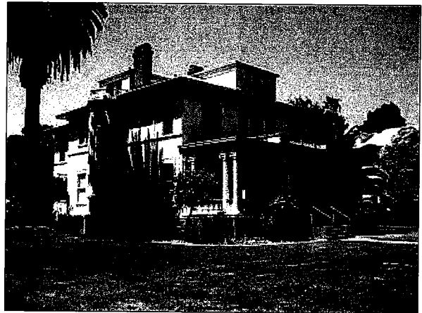
A chimney should be reinforced and/or secured to the structure to minimize earthquake damage to the chimney. Building N
