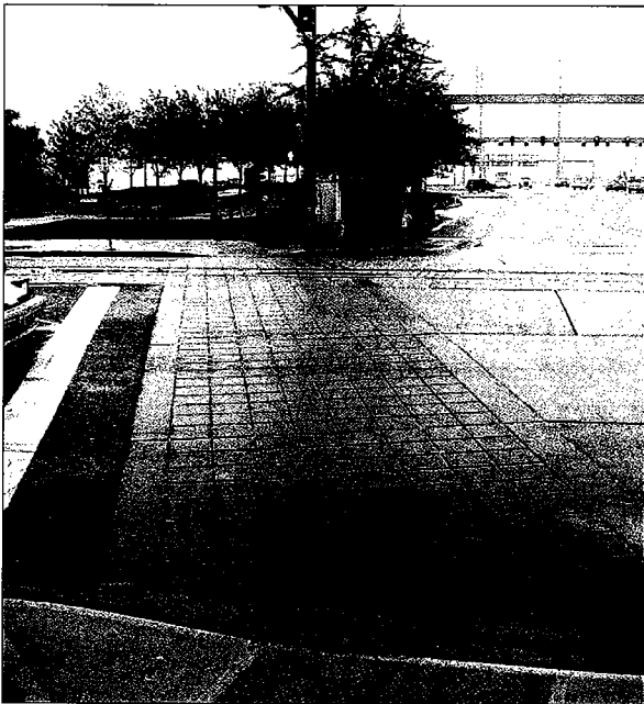
Textured paving, which is muted in appearance, may be considered to define a crosswalk. (Tacoma, WA)
