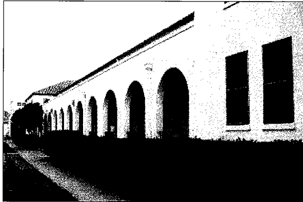
Porches and porticoes should be preserved. This arcade, for example, is a distinctive feature that should be maintained.
