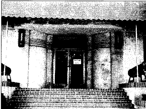
Awning and canopies should be in character with the historic property. This fabric awning is out of character and obscures key features.
