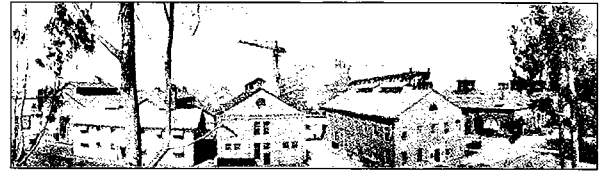
Historic contributor buildings in the Shipyard (Photo: National Archives and Records Administration)
