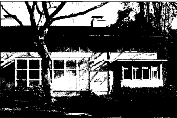
Original window arrangements on key facades should be preserved.
