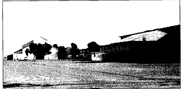
In some portions of the Industrial Character Areas, buildings have large open spaces around them. Historically, these were used for outdoor storage and "laydown" functions. This provides precedent for parking lots. Note also the short row of trees along the edge of the site in the background.
