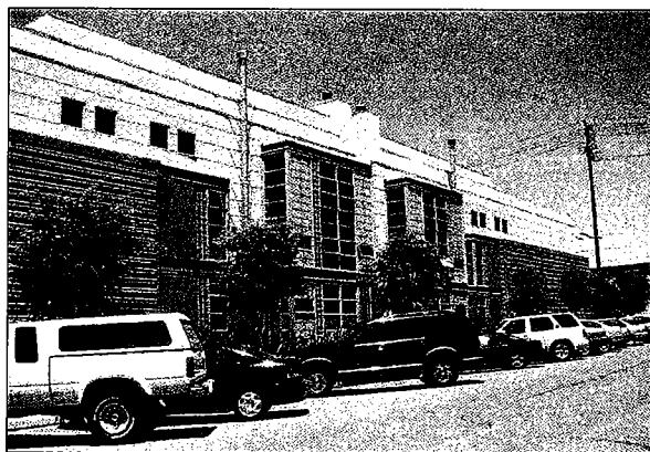
Varying wall planes to create a sense of scale, while maintaining an overall simplicity of form, is appropriate. (Berkeley, CA)
