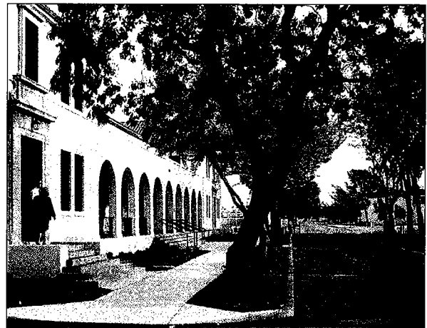
Many sidewalks are detached from the curb.
