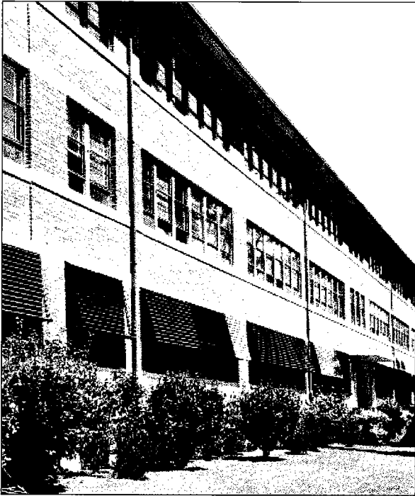
This distinctive awning design relates to the modernist character of Building 521. Reconstructing a feature such as this would be appropriate. (Photo: 1947, National Archives and Records Administration)
