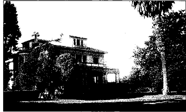
Larger single family houses have one-story porches that provide a consistent scale along the street.
