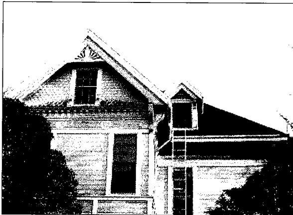
The asymmetrical composition of roofs is a distinct feature of Building M5 that should be maintained.
