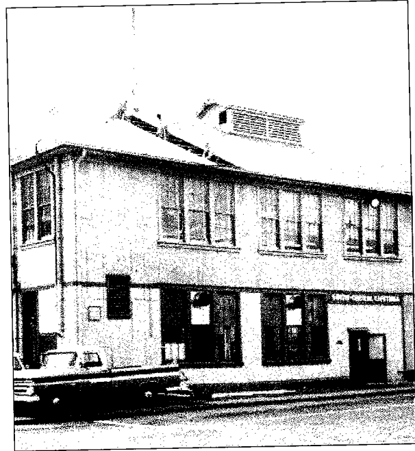
Roof repair (Photo: Building 207/208, 1966, National Archives and Records Administration)
