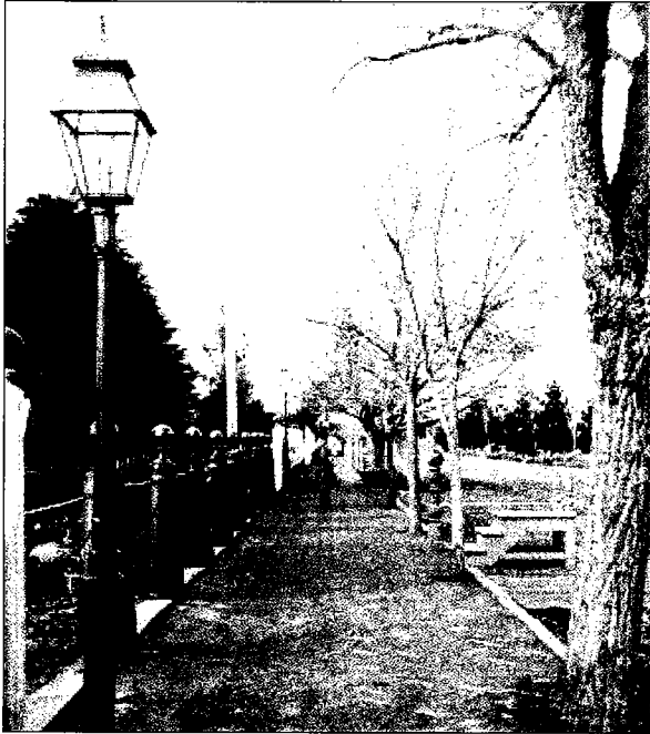
Streetscape designs have changed over the years on Mare Island. In this 1884 image of Officer's Row, brick paving was laid in a herringbone pattern. A "colonial" lamp was used and bollards lined the inner edge of the sidewalk. Street trees were adjacent to the curb. This arrangement was later replaced with a sidewalk that was separated from the curb by a landscape strip or tree lawn, which in itself has taken on historic significance. (See below.) (Photo: National Archives and Records Administration)
