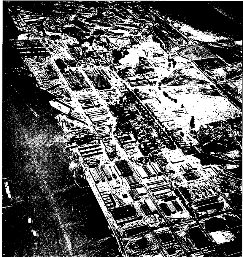
The Mare Island Historic District is dotted with buildings, structures and sites that reflect properties associated with a wide range of military missions, including shipyards, a major naval hospital, a Marine barracks and, during the 20th century, a submarine base. (Photo: c. 1963, National Archives and Records Administration)
