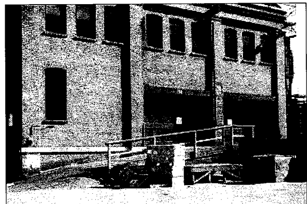
Loading docks and other historic features which convey a sense of the historic character should be preserved. (Building 114)
