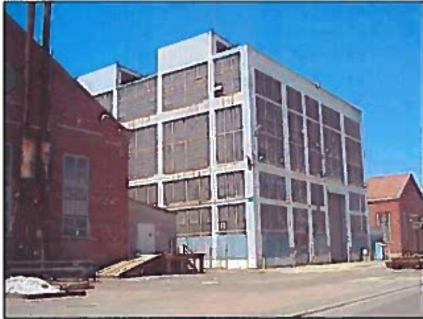
M – Masonry Industrial Shops (Building 0271)
