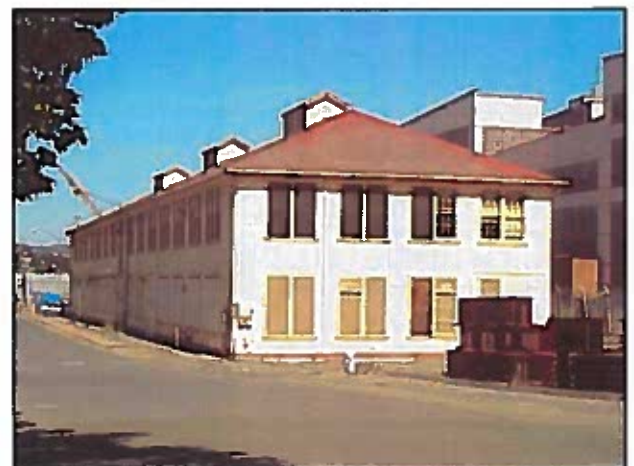
R – Metal-Clad Administrative, Institutional, Or Commercial (Building 0208)
