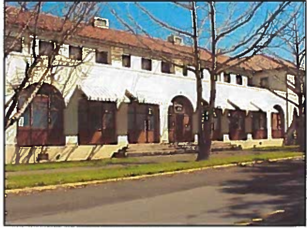
D – Barracks (Building 0459)
