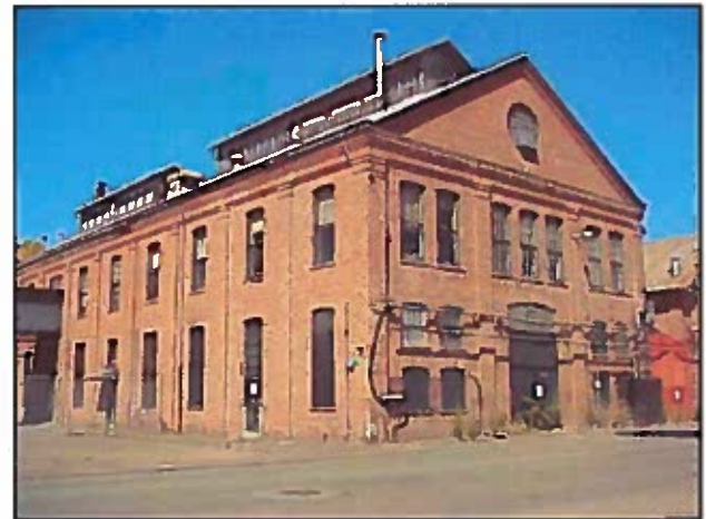
P – Masonry Administrative, Institutional, Or Commercial (Building 0065)
