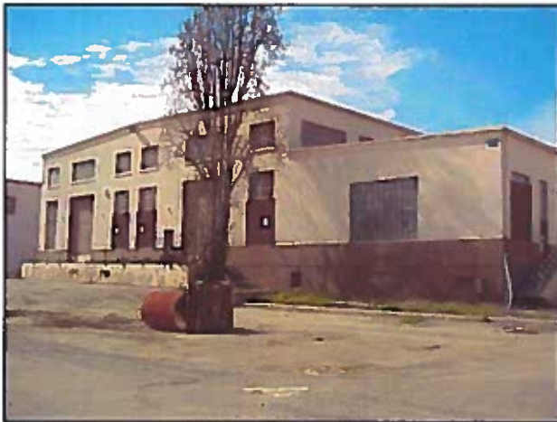
M – Masonry Industrial Shops (Building 0461)
