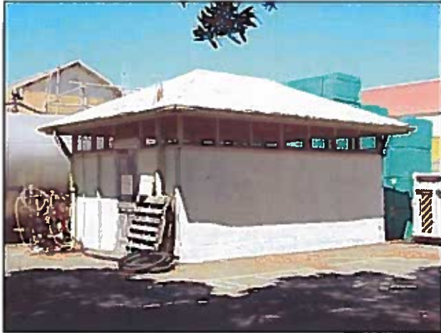
G – Latrine (Building 0077A)
