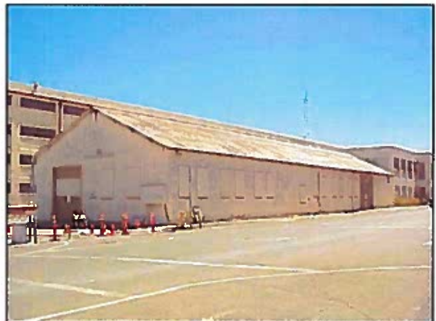
O – Metal-Clad Industrial Shops (Building 0115)
