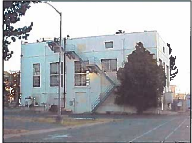
H – Other Infrastructure (Building H074)
