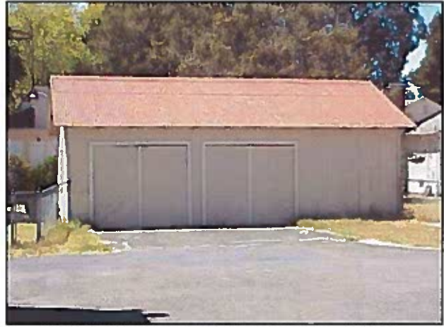
B – Residential Garage / Shed (Building 0133B)
