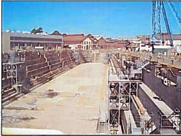
S – Berths/Quays/Causeways (Dry Dock 2)
