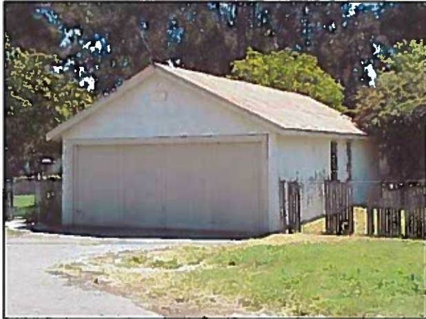
B – Residential Garage / Shed (Building G-B)
