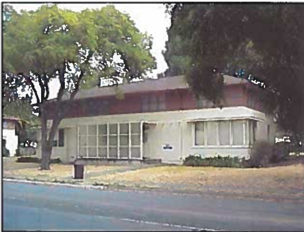
C – Duplex And Multi-Family Residential (Building Q07/08)
