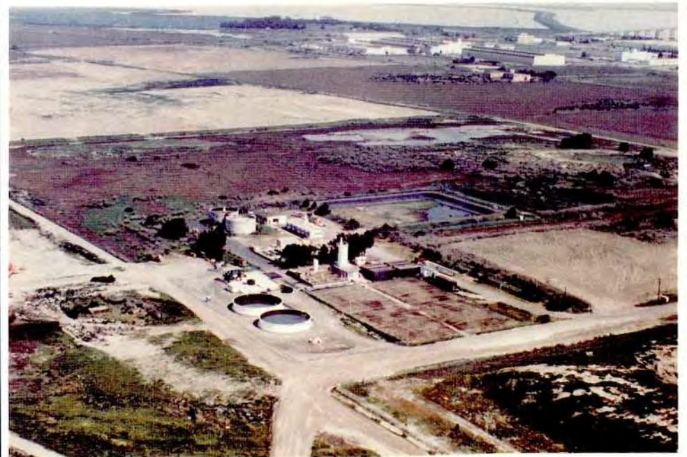
Photo 13: Reuse Area 13 (Recreation/Open Space) showing the waste treatment facility.
