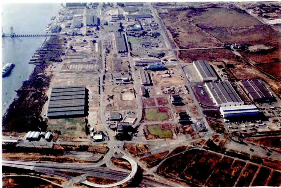
Photo 1: Reuse Area 1 (Light Industry) looking south from Highway 37.
