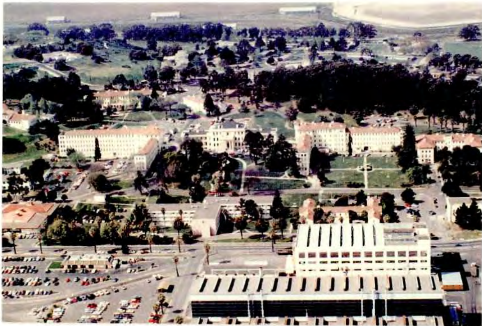
Photo 8: Reuse Area 9 (Educational/Office) looking west.
