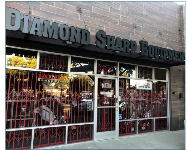
ENCOURAGED: Interior decorative security grille can be folded away when not in use.
