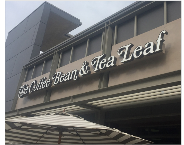
Sign with exposed raceway painted to match background wall.
