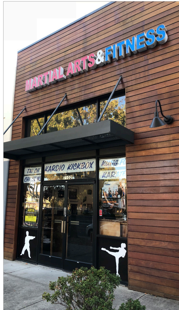
Example of major improvements include updates to: signage, canopy, light fixtures, storefront system, and façade cladding.
