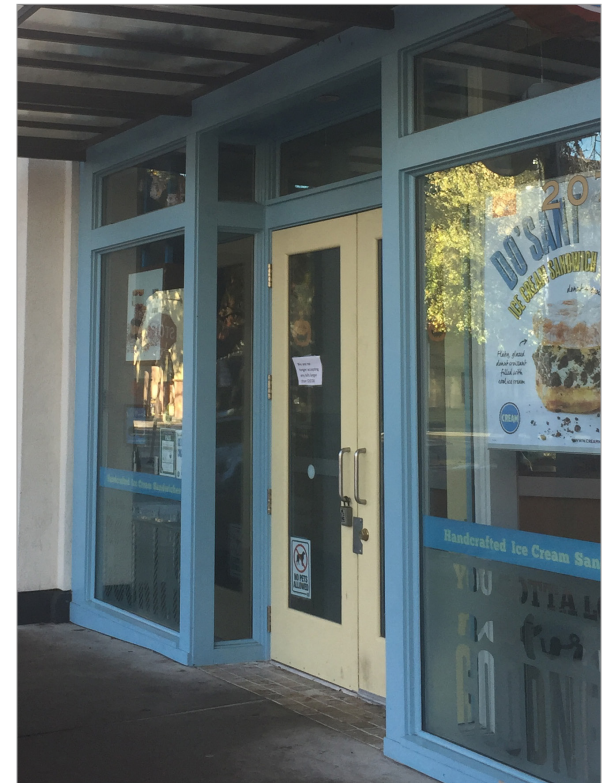
Recessed building entrance protects customers from the weather and prevents doors from swinging open onto sidewalk.
