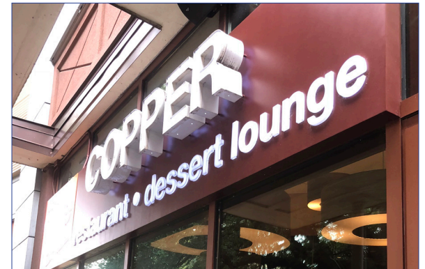
Sign with letters individually pin mounted and illuminated internally.
