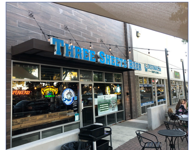
Example of moderate improvements include updates to: signage, canopy, and façade cladding.
