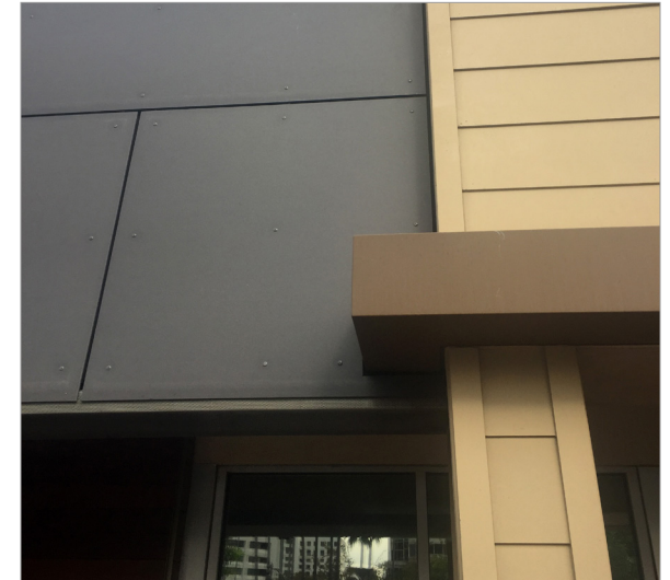
Façade detail of quality materials and the seamless transitions between the materials.
