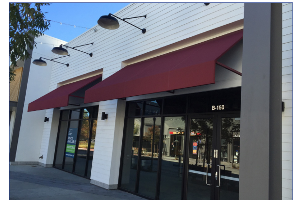
Recessed windows, awnings and decorative lighting help to frame an existing tenant space.
