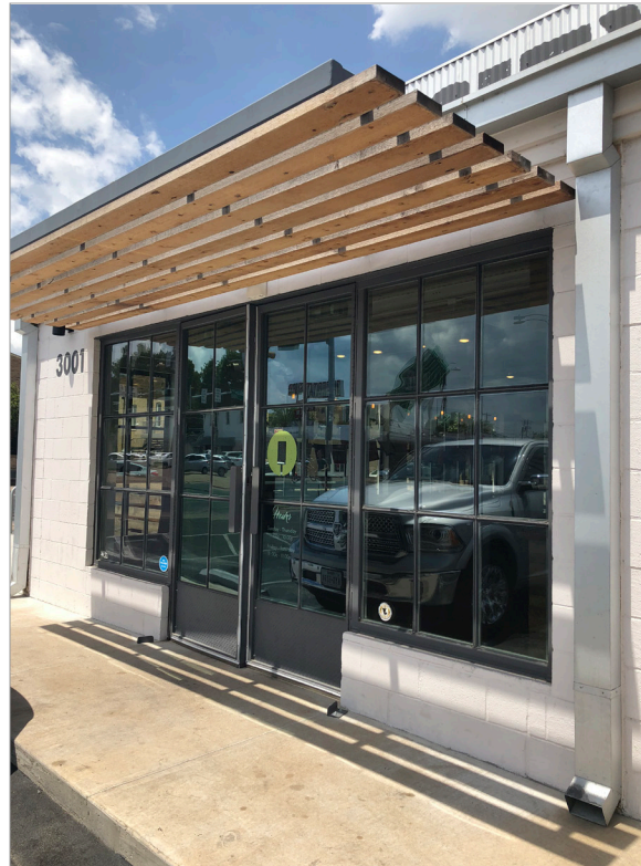
Creative canopy above a primary entrance complements the façade.
