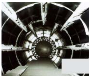
Complete lining with Trellex Granuflex.
